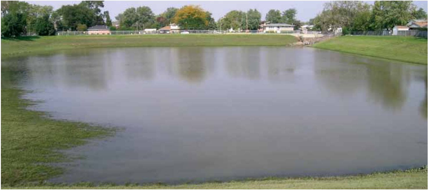
The Melvina Ditch Reservoir after a storm. The reservoir provides flood protection in the Cal-Sag watershed.
