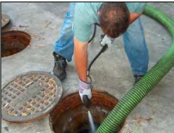
A trap is a small reservoir built into the wastewater piping a short distance from the grease producing area. Baffles in the reservoir retain the wastewater long enough for the grease to congeal and rise to the surface. The grease can then be removed and disposed of properly.
